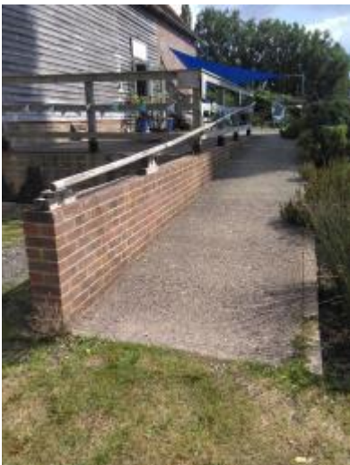
Ramp from car park to reception desk in Farleys Gallery
