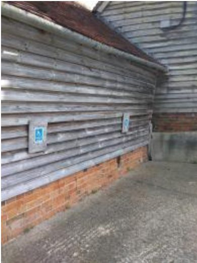
Parking spaces reserved near main entrance to Farleys Gallery
