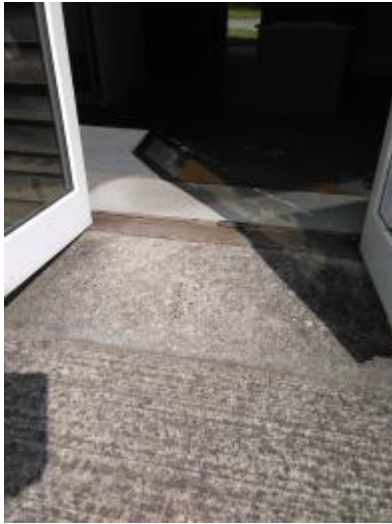
Door to Farleys Gallery from car park
